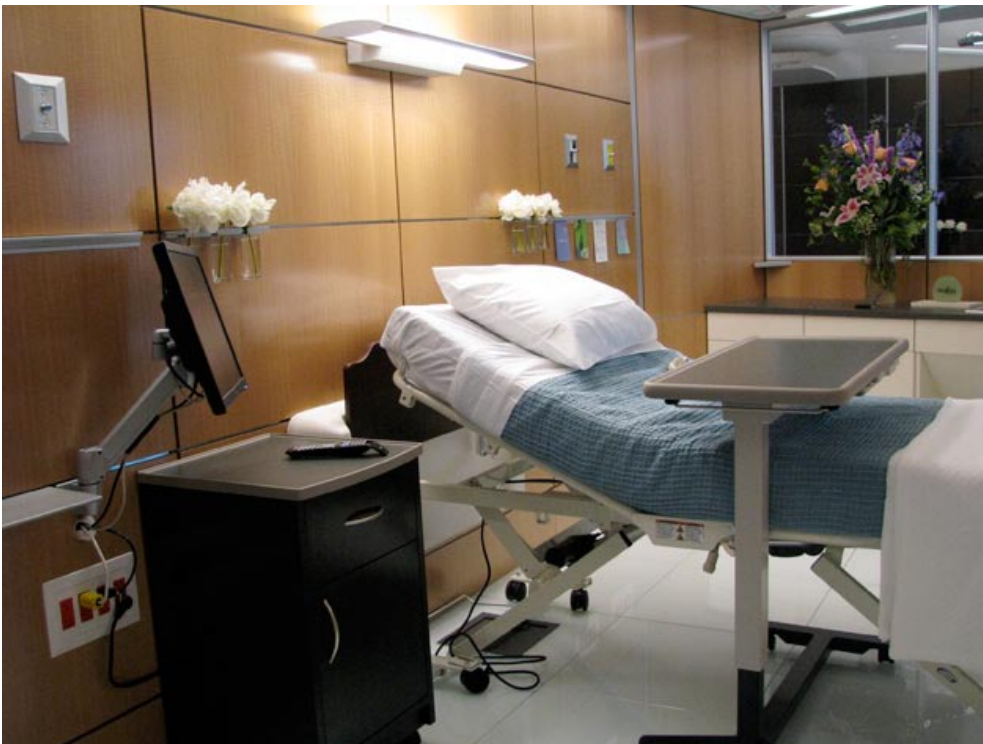
DIRTT WALLS IN A PATIENT ROOM
